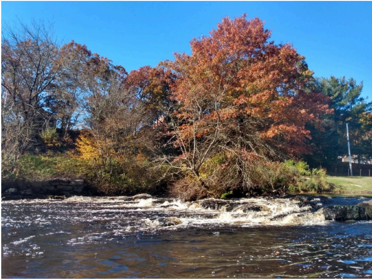
BROKEN DAM ON THE PAWCATUCK RIVER NEAR BURDICKVILLE ROAD (PHOTO BY DAN NELSON)
